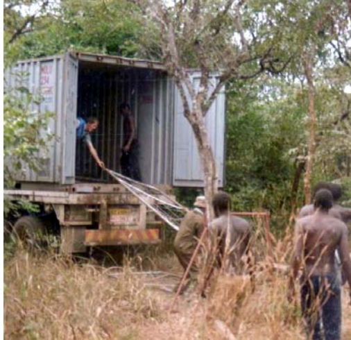
Building material being offloaded
