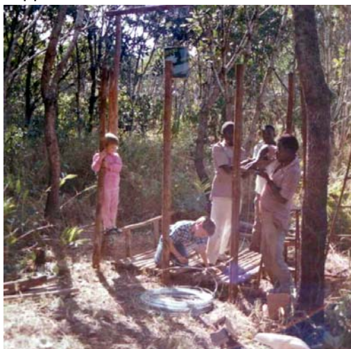
The new shower at Mzuzu station
