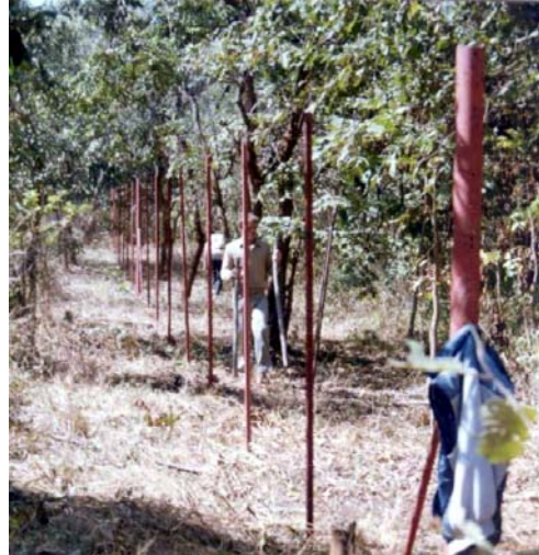
Construction of two quarantine stations
